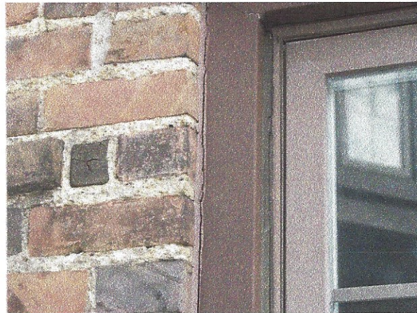
Sealant crack
