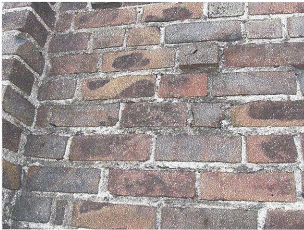
Typical mortar deterioration
