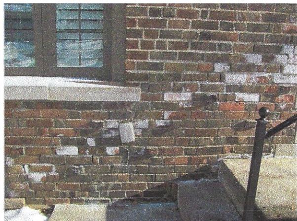
Efflorescence
