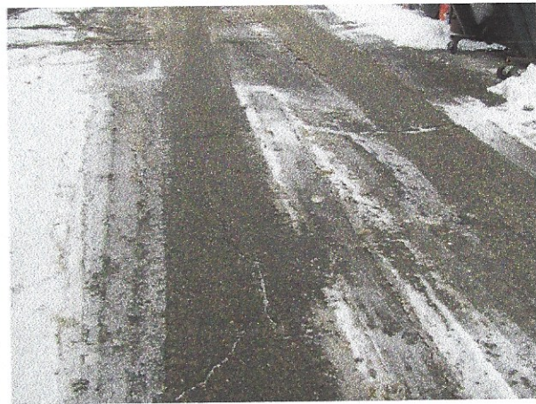
Cracks and settlement evident at asphalt pavement
