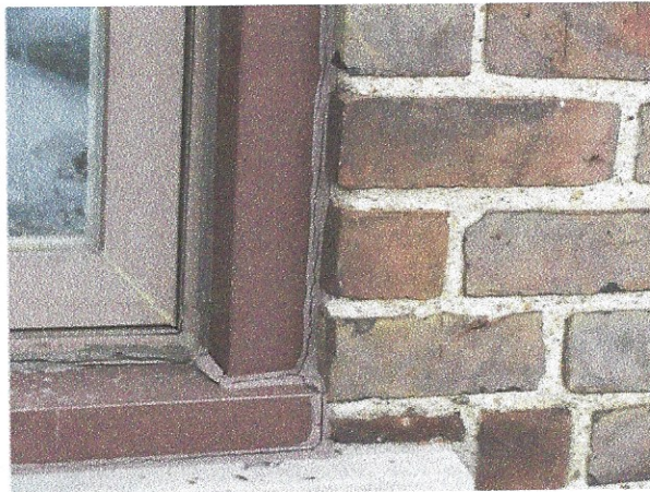
Sealant cracks
