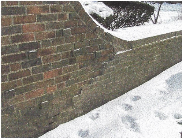
Step crack and movement evident at front perimeter wall
