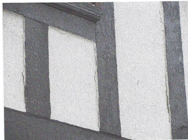
Stucco deterioration at wood interface
