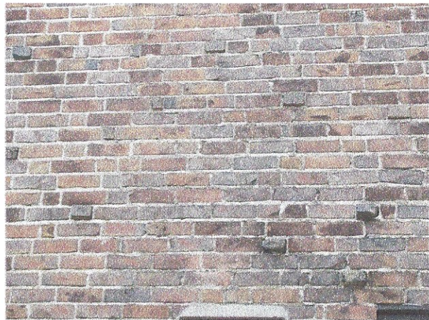
Typical mortar deterioration
