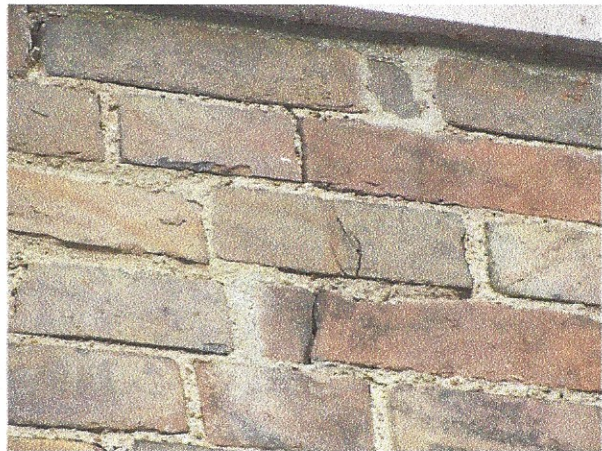
Masonry cracks
