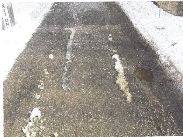
Potholes and deterioration
