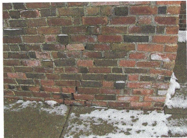
Previous repairs and recurring deterioration at storage room
