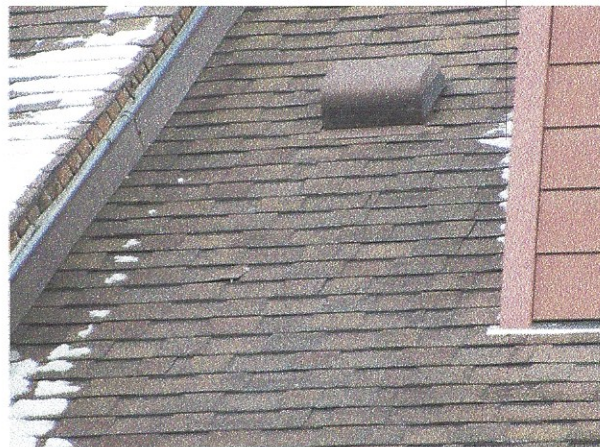
Granular loss at shingles
