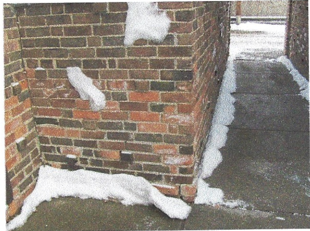
Spalled and deteriorated masonry at garage
