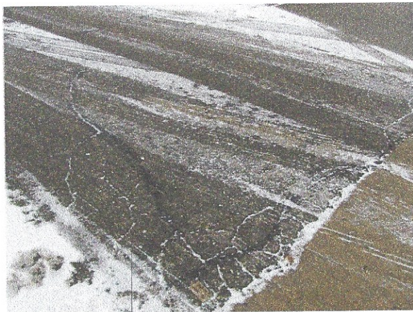
Alligator cracks
