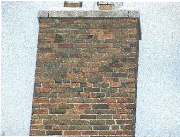
Mortar deterioration and previous repointing evident
