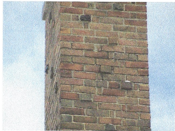
Mortar deterioration
