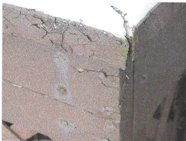
Wood deterioration and popped nails evident
