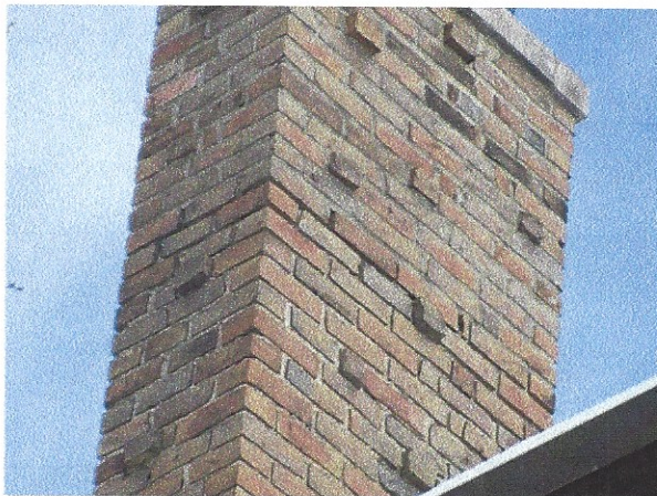
Significant area of mortar deterioration near middle
