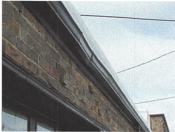
Damaged gutter at garage
